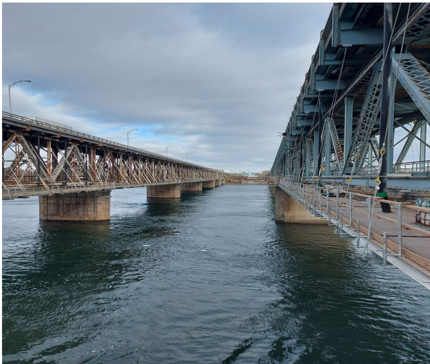
Suspended platform - Mercier Bridge
