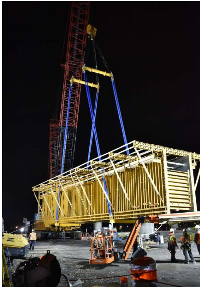
EFCO double plate girder lifting
