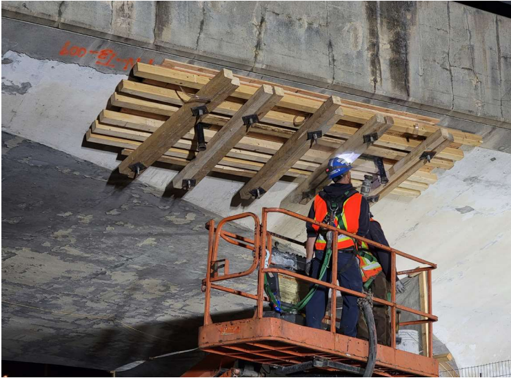
Formwork for tunnel repair
