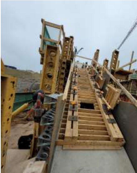
Inclined formwork
