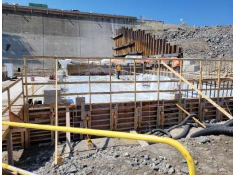
Slabs, raft foundation and foundation works
