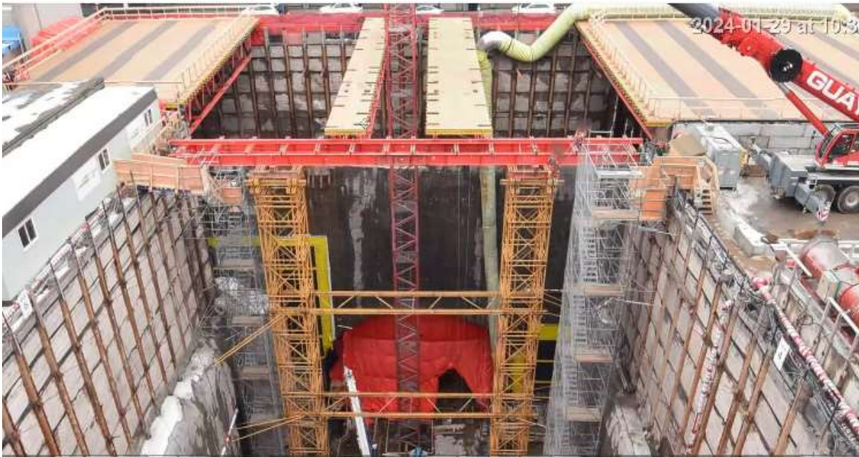
Winter protection structure PERI variokit Truss and EFCO shoring towers
