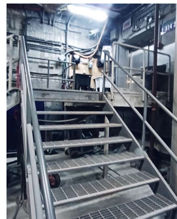
Emergency stairs compliance upgrade
