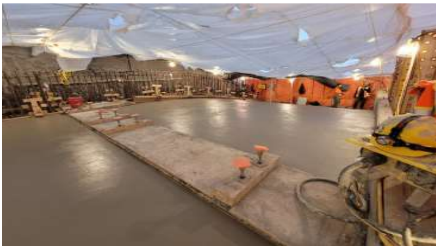
Special pours and winter protection structure
